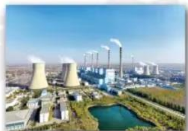
Electric Power Plant
